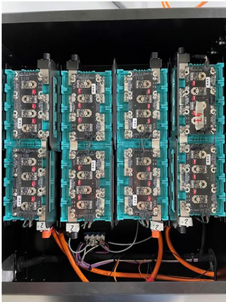
HV battery of the control and power supply module
